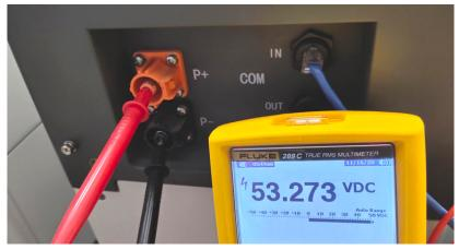
The voltage measured on the PDU is the average voltage of all modules in the tower and should be around 50V. NOTE: the PDU output voltage will only be correct if the battery has been configured correctly via app and then restarted. Without correct app configuration, the PDU output voltage will be wrong!
